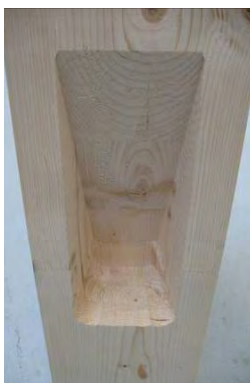
Fig. 1: Notch type shear connector.
