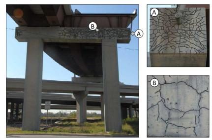
Figure 1: Typical Field Damage (US-59 and I-10 Interchange in Houston, Texas)
