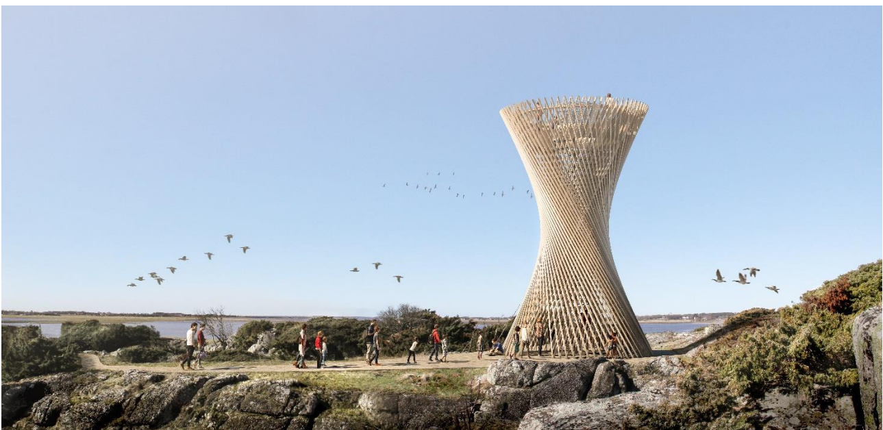
Figure 1. Competition entry rendering of The Sheaf, a hyperboloid timber-diagrid lookout tower.
