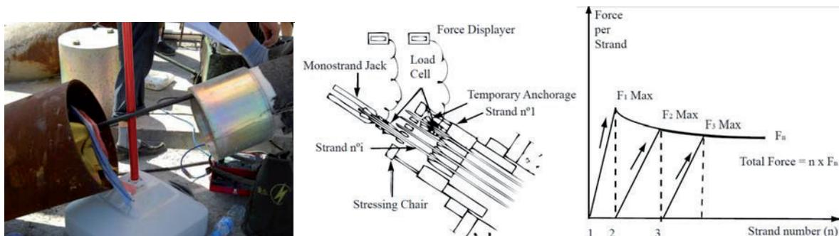
Figure 2. (A) Multi-strand stay cable, (B) Technology of the Isotension method and (C) Isotension principle diagram.
