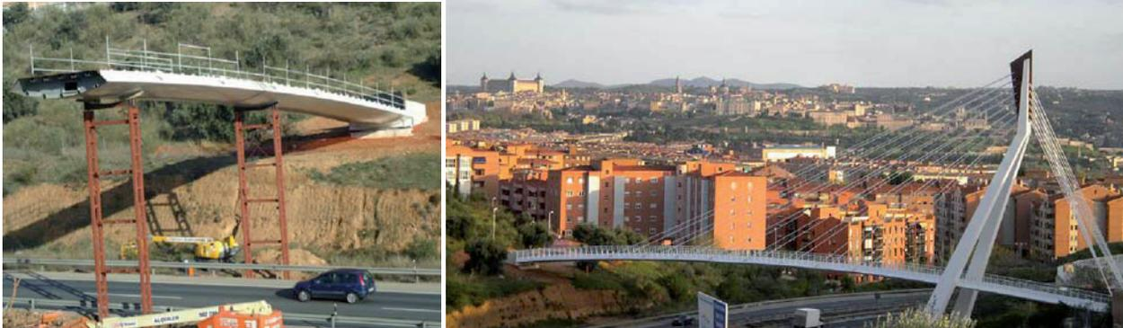
Figure 1. Cable-stayed footbridge in Toledo (Spain) built on temporary supports. (A) Deck erected on temporary supports and (B) Finished structure or OSS. Pictures of Ramón Sánchez de León (AIA)
