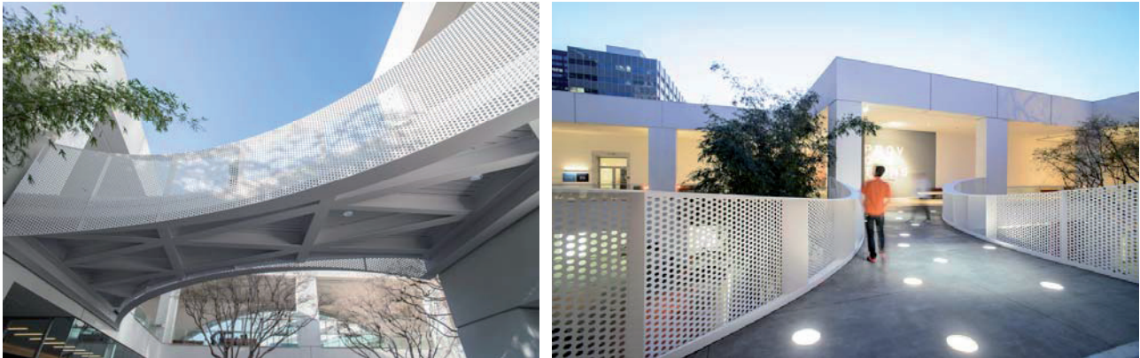
Fig. 1. and 2. The John V Tunney Bridge at the Hammer Museum (Photos by MMA)
