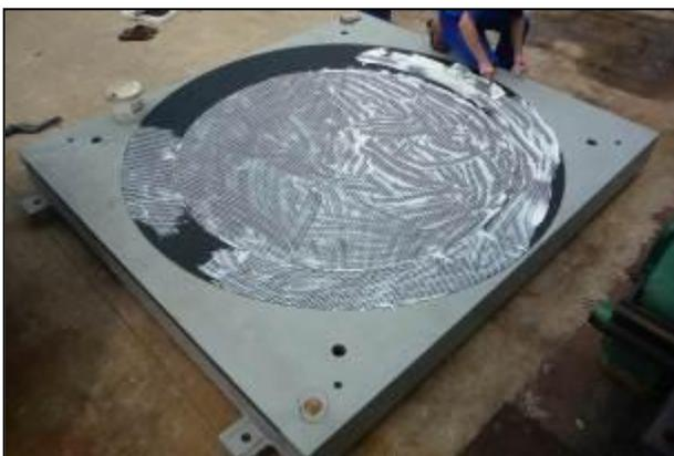
Fig. 1: Lower bearing part during application of special silicone grease to sliding material
