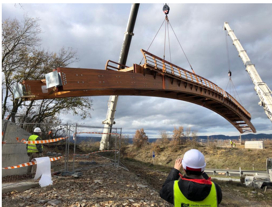
Fig. 1. One-step erection process for the timber footbridge.
