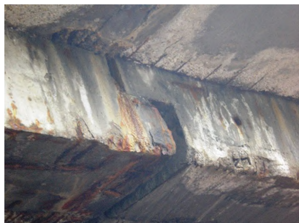
Figure 1. Gerber joint of RC bridge in Sofia, 2008
