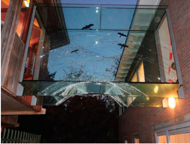
Fig. 2, A broken but still functioning glass bridge.
