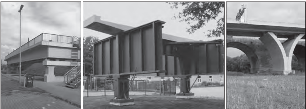
Fig. 3: Attempts to deal with the motorway bridge-building inheritance: the “Weg Hesseler” prestressed concrete overpass (1938) following its relocation to the Vellern motorway rest area; a preserved segment of welded superstructure from the Mühlenfliess Bridge (1937/1938)—now an exhibit in the motorway history collection at Erkner Motorway Maintenance Depot; the extension (2003–2005) to the Saale valley bridge at Jena (1938–1941) with an “appropriate” design language
