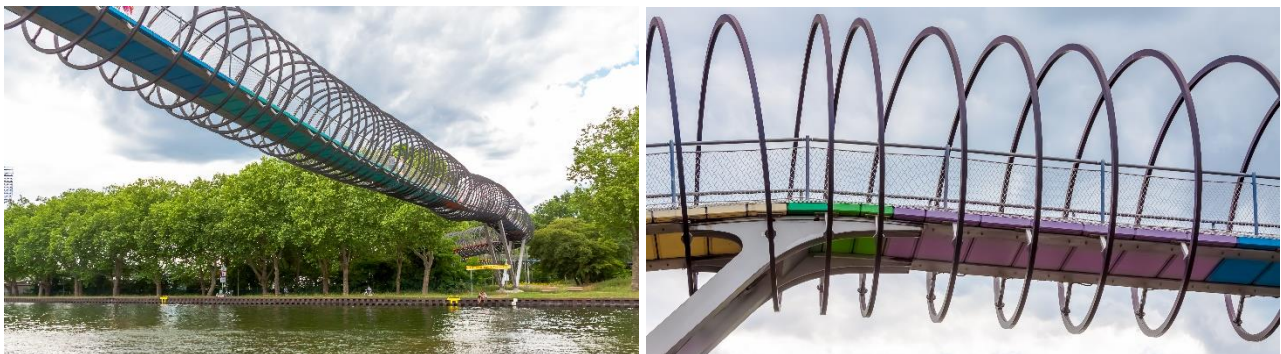
Fig. 1. Stress ribbon bridge Slinky Springs to Fame in Oberhausen / Germany (photo: Christoph Hasler)
