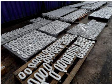
*Fig. 3. Dismantled bridge elements labelled and painted in workshop*
