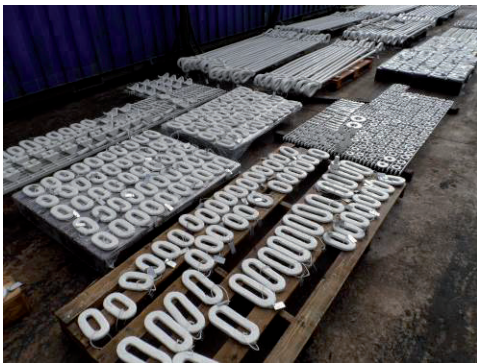
Fig. 3. Dismantled bridge elements labelled and painted in workshop
