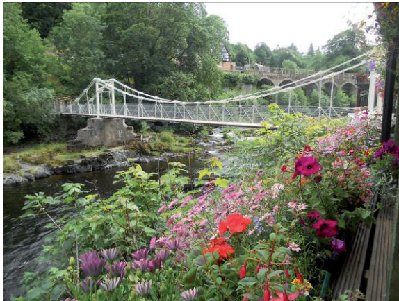
Fig. 1. Complete Bridge viewed from downstream on the Hotel North Bank
