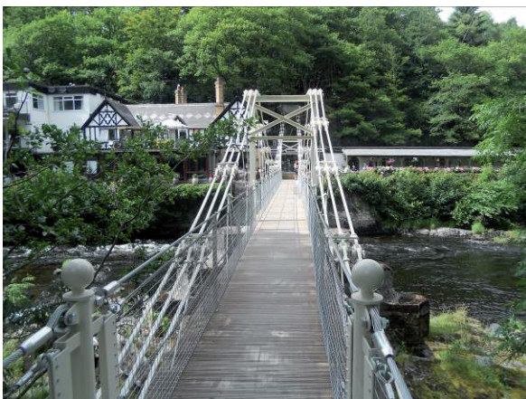
Fig. 3 Complete Bridge viewed from the south bank
