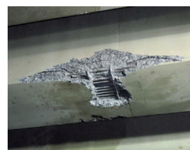
Fig. 1: Damaged area of inner beam
