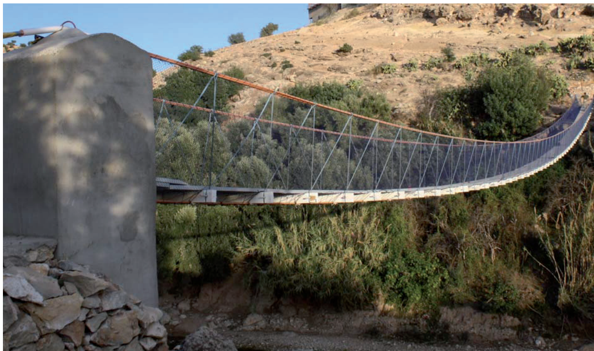
Fig. 1. Realized 64 m span polyester-rope suspended footbridge in Ait Bayoud, Morocco
