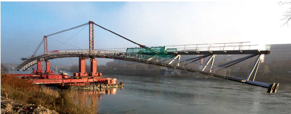
Fig. 2. Temporary suspension system and pontoons, Photo by Michael Zimmermann
