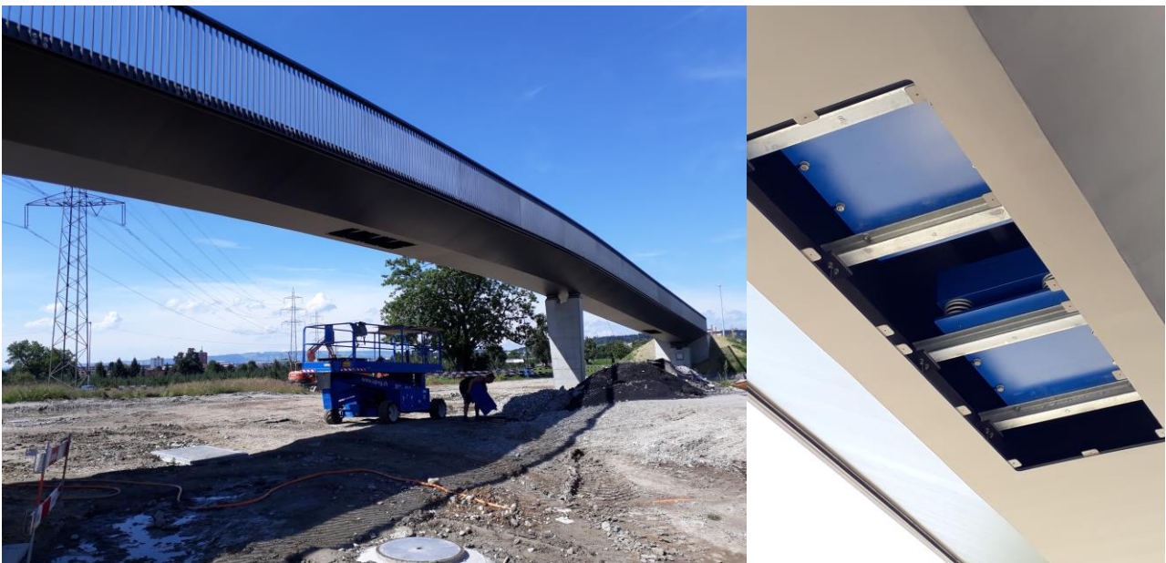
Fig. 1. Footbridge "Inwilerstrasse" near Zug in Switzerland (left) and installed TMDs (right)
