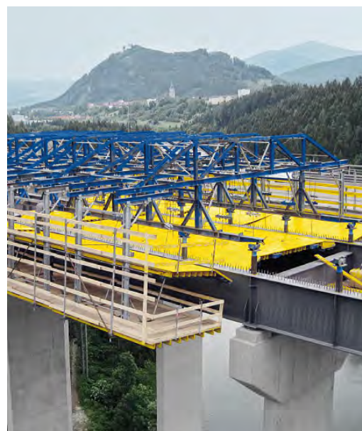
Figure 1. Formwork carriage (photo: DOKA) [1]
