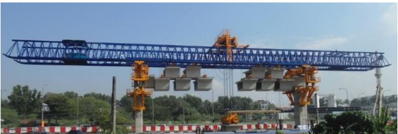
Figure 0: Hybrid Launching Gantry used in LRT Kelana-Jaya Line Extension Project Package-A
