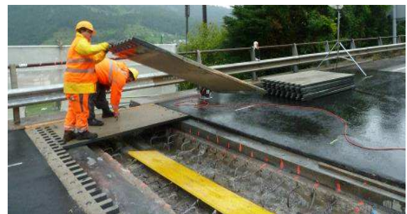
Figure 1. Placing of Mini-Fly-Over plates to allow traffic to cross an expansion joint replacement worksite during peak traffic periods
