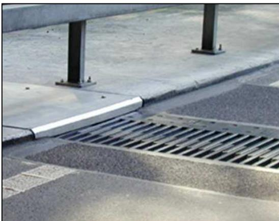
Fig. 1: A Tensa® Flex expansion joint
