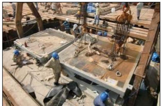
Fig. 2: Placing of two enormous guided sliding spherical bearings, side by side to support pylon
