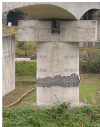
Figure 1. Failure of pier at bar termination zone
