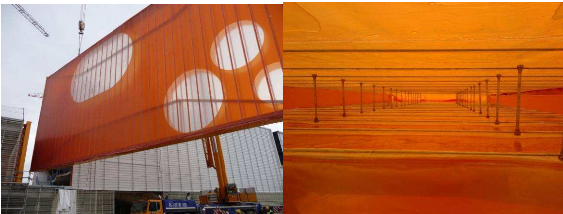
Fig.1: General view of the ETFE membrane during installation and inside view
