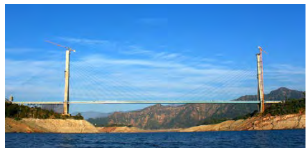
Figure 1. Atal Bridge, 350m cable-stayed span
