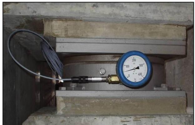
*Fig. 1: The ongoing condition of the Pont Nanin structure in the Swiss Alps has been monitored by an SHM system (with force monitoring at bearings as shown) since its static design was changed a decade ago (fixing one end of deck) [1]*
