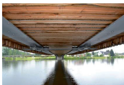
Fig. 8-9. Dynamic absorber, mounted under the bridge
