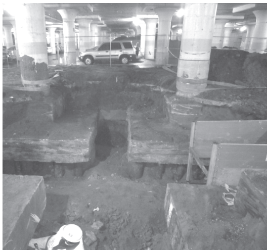
Figure 2. Test pit with exposed pile caps and timber piles
