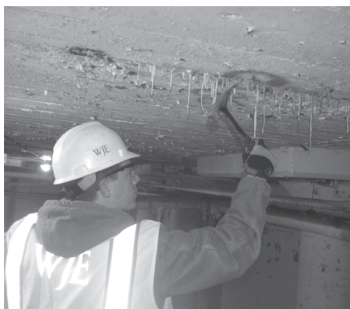
Figure 3. Efflorescence, leakage and deterioration of concrete along construction joint in track deck
