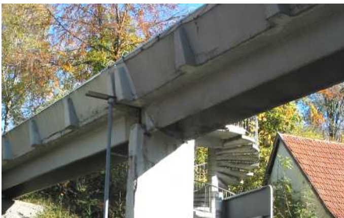
Fig. 1: Former pedestrian bridge in Albstadt, Germany (Photo by Groz-Beckert Group)
