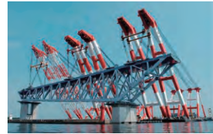
Fig.4: A truss block erection using three floating cranes simultaneously
