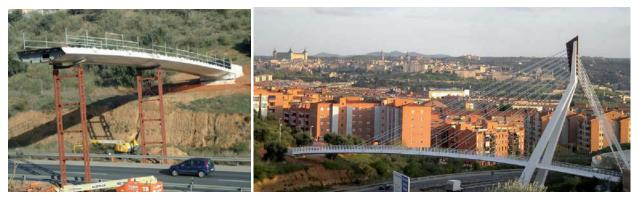
Figure 1. Cable-stayed footbridge in Toledo (Spain) built on temporary supports. (A) Deck erected on temporary supports and (B) Finished structure or OSS. Pictures of Ramón Sánchez de León (AIA)
