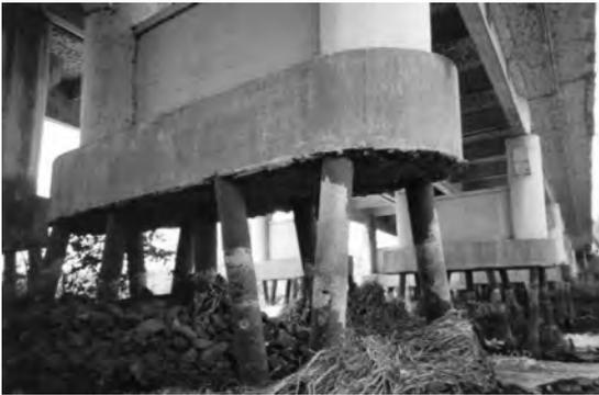
Fig 1–Detail of foundation of a bridge (pile footing and piles exposed)
