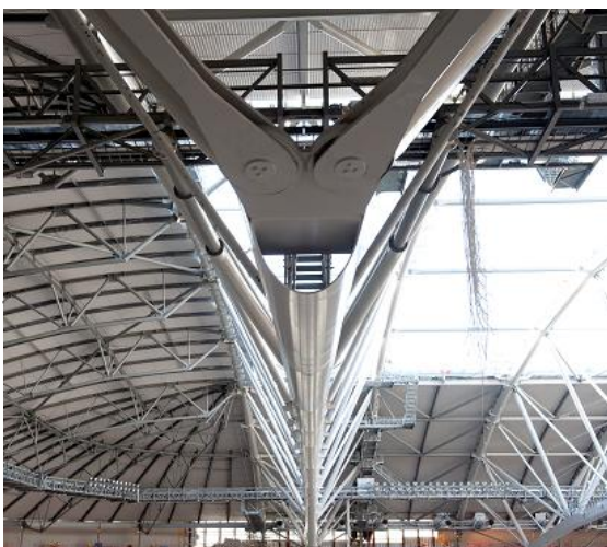
Fig. 1: Friends Arena, Main truss- Bottom chord and tension bars
