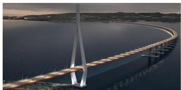
Figure 2. End Anchored Bridge
