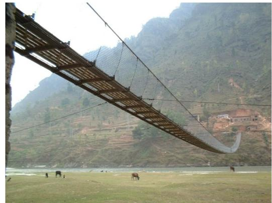
Figure 1: Catwalk or suspended Type
