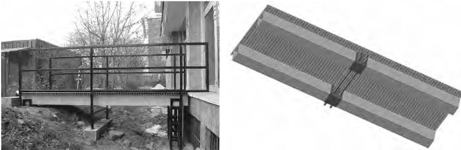
Fig. 3: Research footbridge – phase zero for comparison (main beams without any joints) and Research footbridge – visualization of main beams with joints - bottom view
