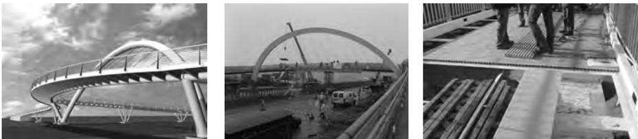
Fig. 4: Visualizations and general view of the complete footbridge Assembling of main span (left) and of composite polymer deck (right)
