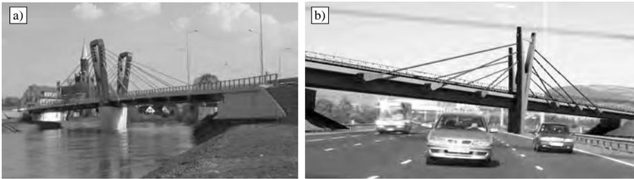
Fig. 1: Curved cable-stayed bridges: a) over the Nysa Klodzka River in Skorogoszcz (after its opening to traffic), b) over the A4 motorway in Wykroty (computer image)
