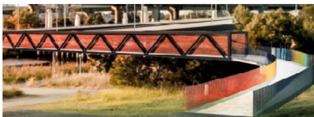
Fig. 1. 60m truss span over Moonee Ponds Creek
