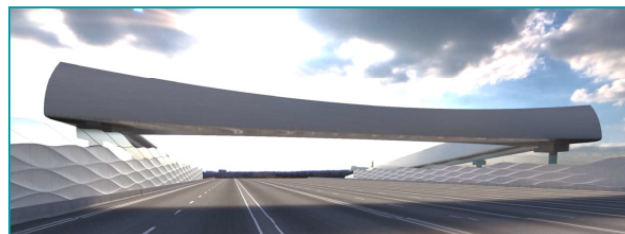
Fig. 2. 70m clad truss over 12 traffic lanes
