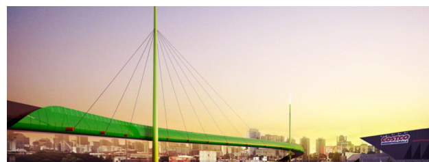
Fig. 4. 120m span cable stay footbridge
