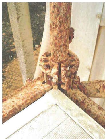
Fig. 1: Deterioration of existing structure with corroded pipes and connectors (detail)
