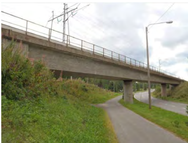
Figure 1. The old box girder bridge
