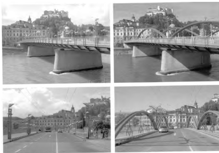
Fig. 1: “Karolinen – bridge” in Salzburg / Austria before (left) and after (right) strengthening
