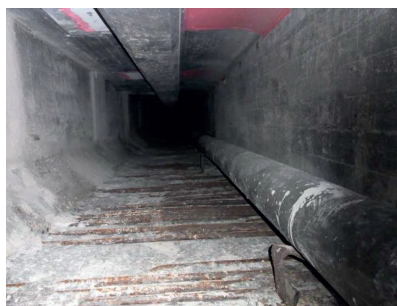
Figure 1. Observed corrosion in the ventilation tubes of the Maastunnel
