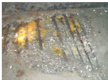
Figure 1. Observed corrosion in the ventilation tubes of the Maastunnel
