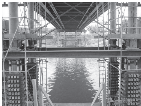
Fig. 3: Raising of the Roosteren Bridge
