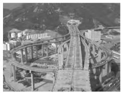
The project is made up of 20 individual bridges, each one separated by a movement joint.
