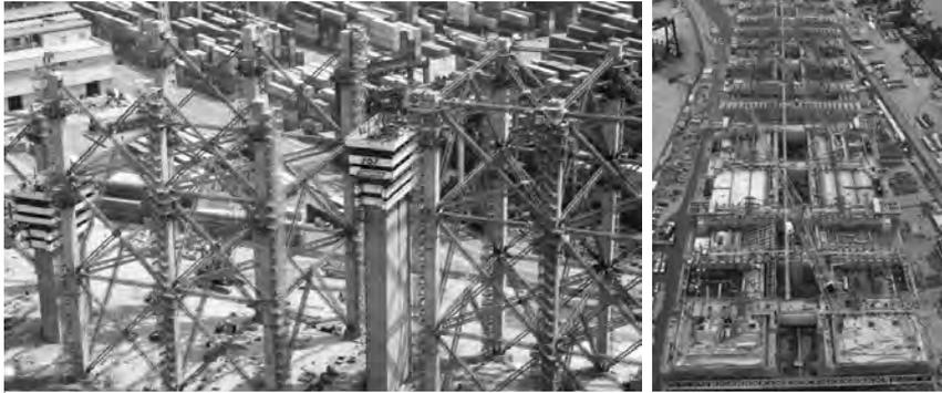
Fig. 1: Falsework erection (left), staged casting of longitudinal girders (right)
