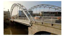
In just 22 months the most important bridge in the city of Bamberg was demolished and replaced by an imposing new one. The view of the new Luitpold Bridge is dominated by a harmonic, rounded steel structure, consisting of three-dimensional truss arches. The harmonious visual aspect of the arch design was achieved by using MSH sections of constant diameter and different wall thicknesses.
